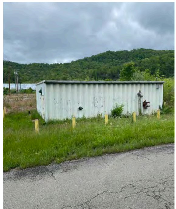
Photo 12- Small metal building found onsite along Industrial Park Road
