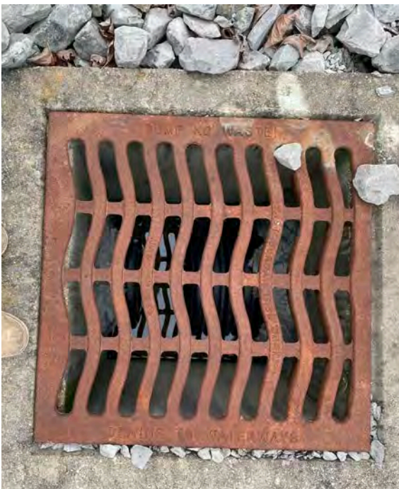
Photo 11- Drain found on the west side of the site that drains to waterways.
